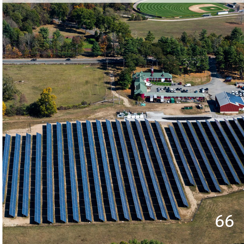
Solar field and rooftop installations at the David Ames Clock Farm at Stonehill College.
